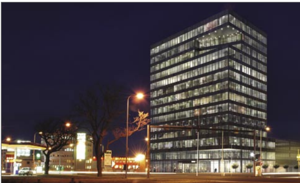
• Delta Plaza - an A-class office building on Tallinn's busy Pärnu Road.
