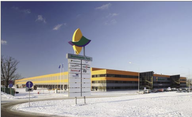
• Dominante Park - the largest industrial park in the Baltic States, on 65 ha on Riga ring road and the A7 highway.
