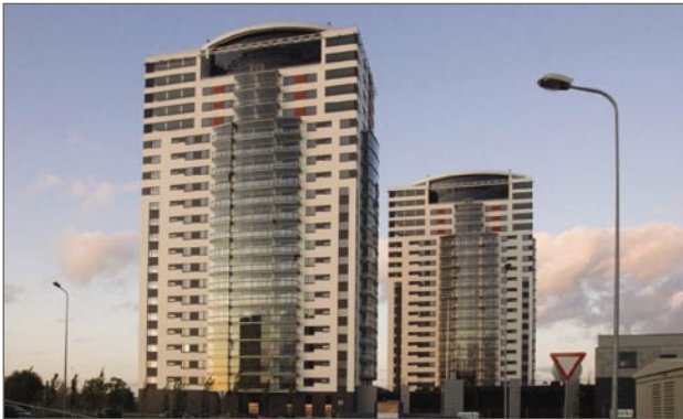
• Skanstes Virsothes - leading Merko Group builds a 75,400 sqm apartment complex near Riga city centre.
