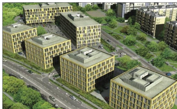
• Malta Office Park; Echo Investment S.A.
