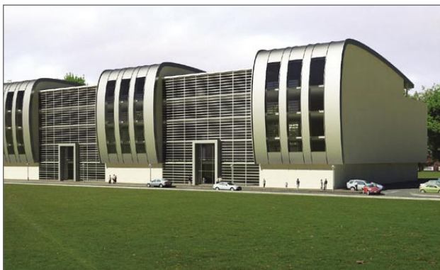
• Alstar Office Center
