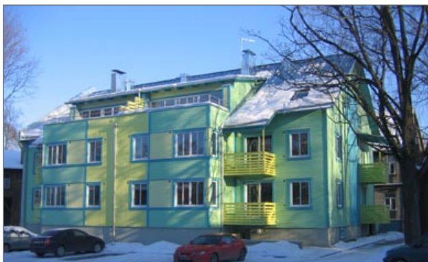
• Tartu, South-Estonia, Kroonuaia - new apartment houses next to city centre. Developer Eleven EST OÜ.
