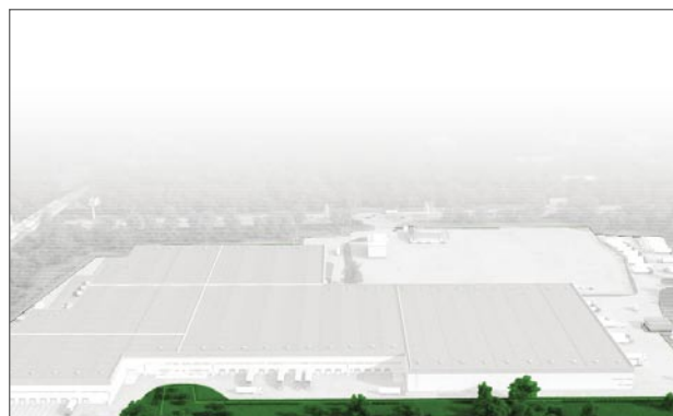
• Comodor Logistics Park, modern, hi-tech commodious office, warehouse and logistics centre.
