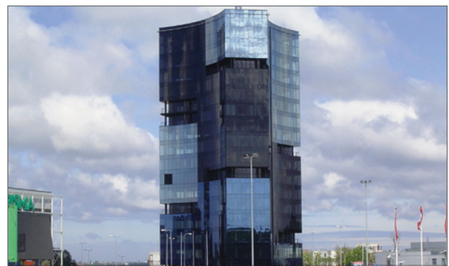
• Al Mare office building, one of the first new office buildings in Öismäe area, developed by Ühendatud Kapital.
